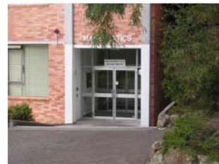
Entry from the Central Mall
