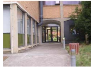
Entry from Clark Road
